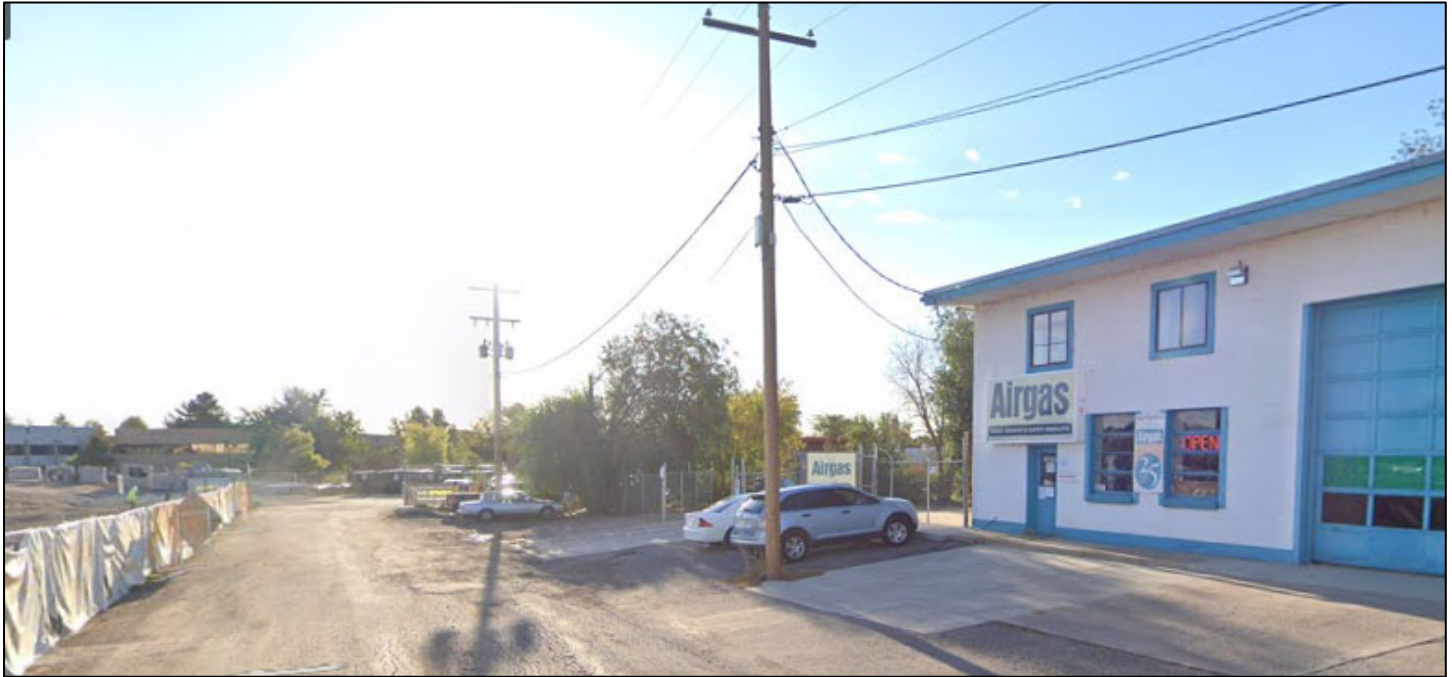
Figure 44: Overhead Utility Lines on Bluff Street Near Proposed Boulder Junction at Depot Square Station
