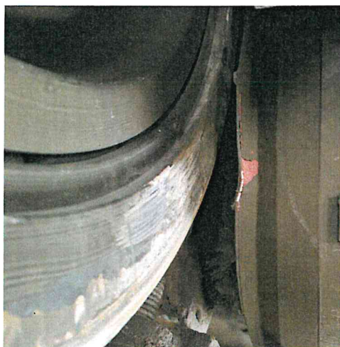
Image 24: Damage on tank
