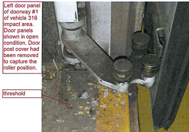
Image 16: Lifted out roller swing arm
