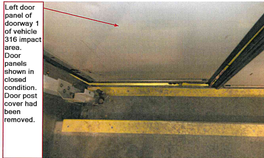
Image 7: Stairs at door 1
